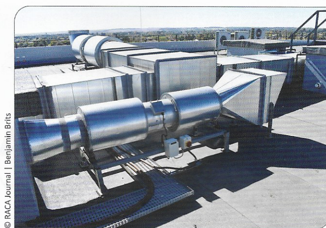
Roof plant – typical bedroom bathroom extract system.
