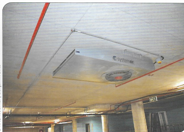
Basement level – typical jet fan installation for day-to-day and smoke extraction.
