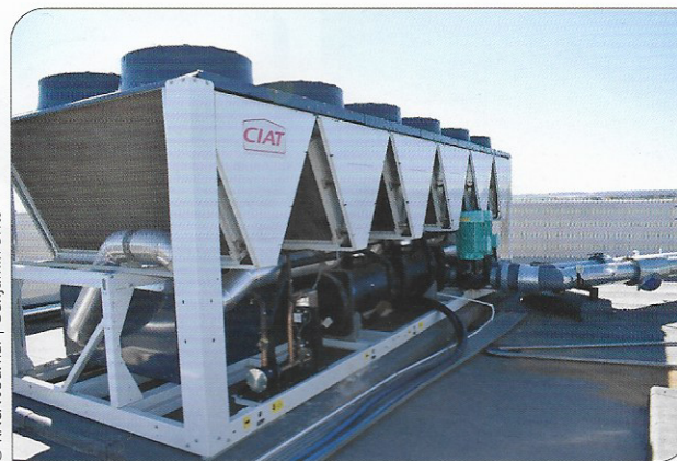
Roof plant – chilled water generators.
