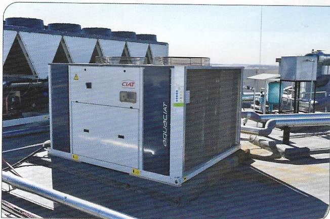
Roof plant – chilled water generators.
