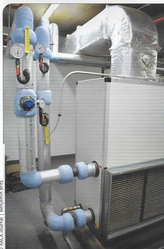
Typical chilled water air handling unit installation.
