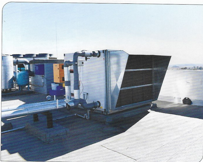
Roof plant – tempered fresh air unit.
