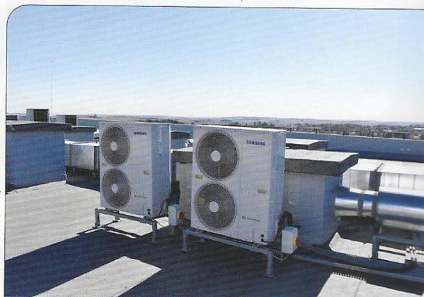
Roof plant – a typical DX unit.
