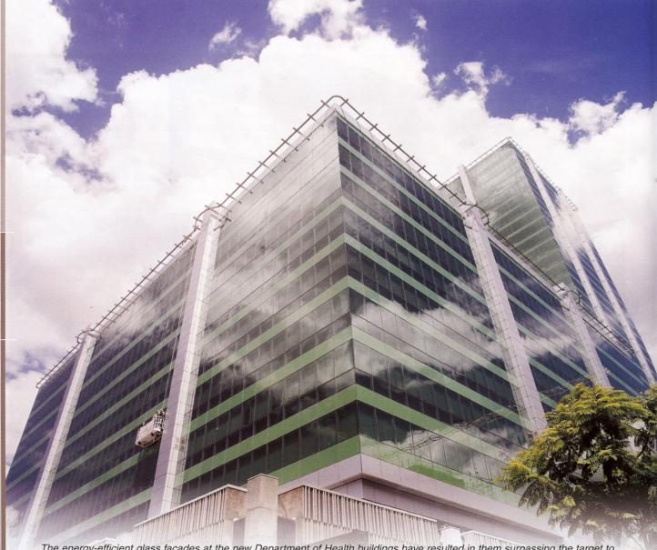
The energy-efficient glass façades at the new Department of Health buildings have resulted in them surpassing the target to reduce overall energy consumption by 24% on the air-conditioning scale of consumption
